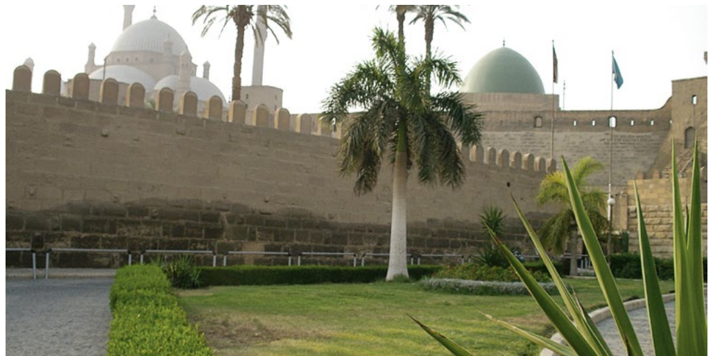
Example of rising damp
