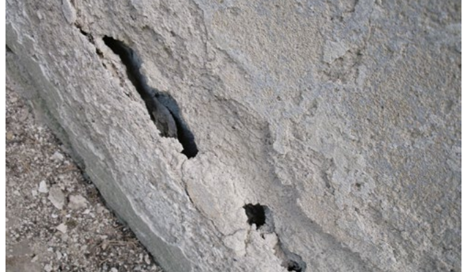
Damaged plaster
